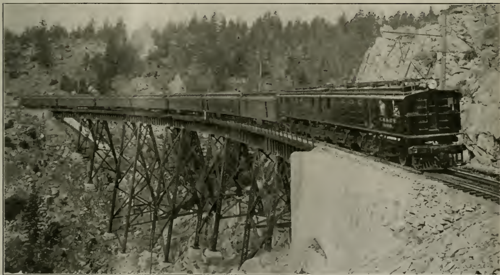
CHICAGO, MILWAUKEE AND ST. PAUL, 3,000 V. D. C. ELECTRIFICATION TRAIN NO. 16 DESCENDING 2 PER CENT GRADE.
